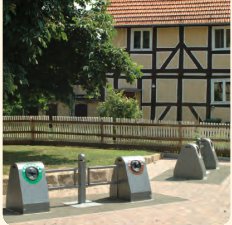
Central depot container – underground collection site
